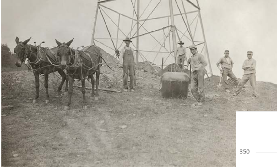
AEP Archives – 1925 Backfilling crew on tower construction on the Philo-Canton transmission line in Ohio
